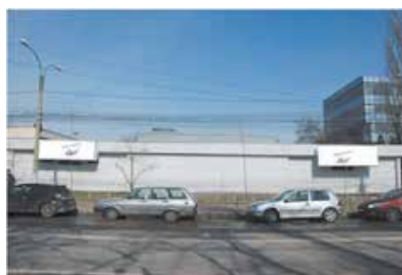
BANNER DISPLAY ON ROMEXPO HEADQUARTER FACADE
