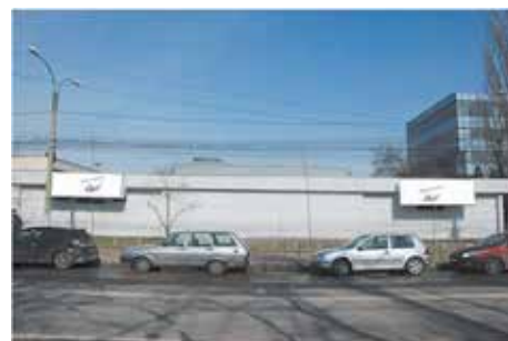
BANNER DISPLAY ON ROMEXPO HEADQUARTER FACADE
