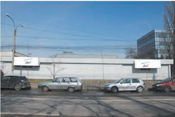
BANNER DISPLAY ON ROMEXPO HEADQUARTER FACADE
